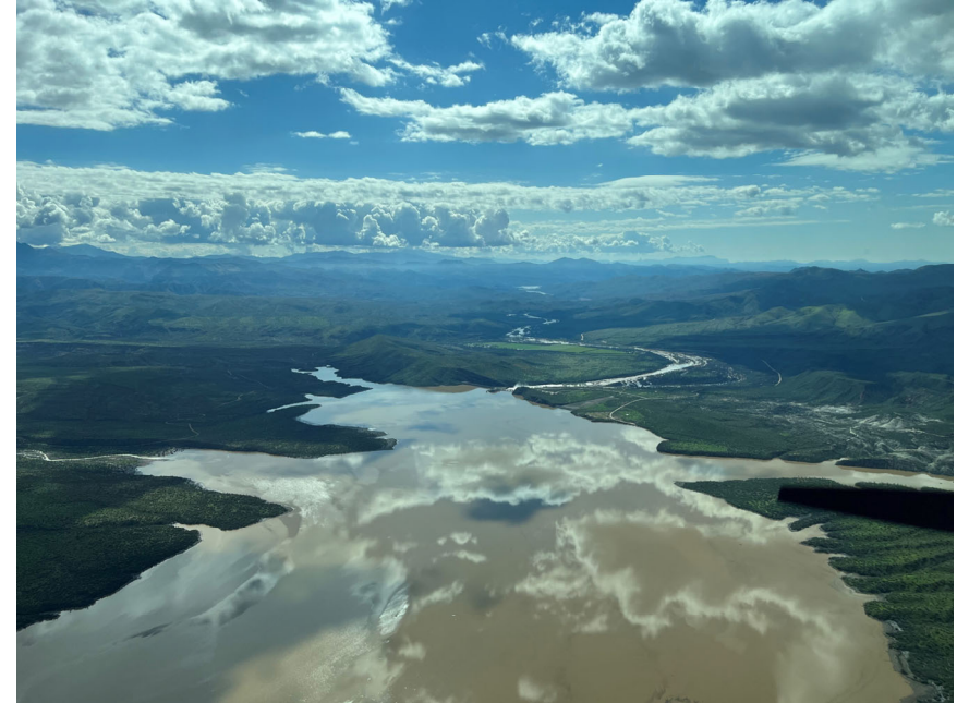
Horseshoe Reservoir 90% full looking south (March 17, 2023)
