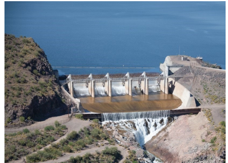
Horseshoe Dam Reservoir and Spillway
